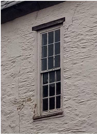
Figure 13: A window on the southeastern elevation in poor repair
