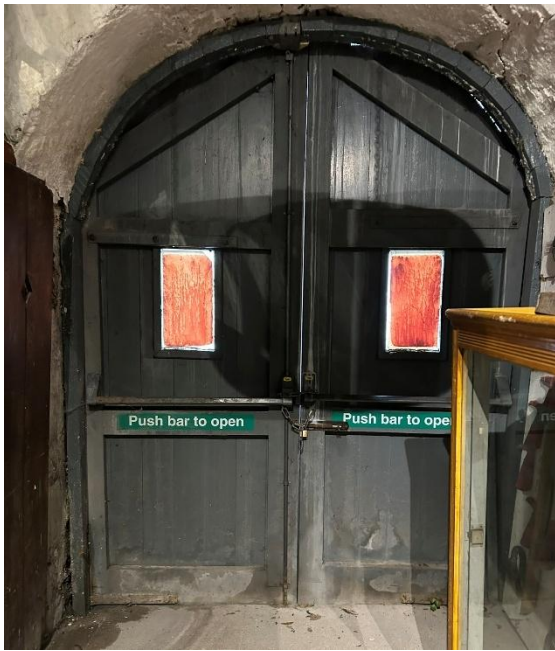
Figure 24: Internal view of fire doors
