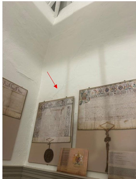
Figure 12: Internal cracks which correspond to the external cracks
