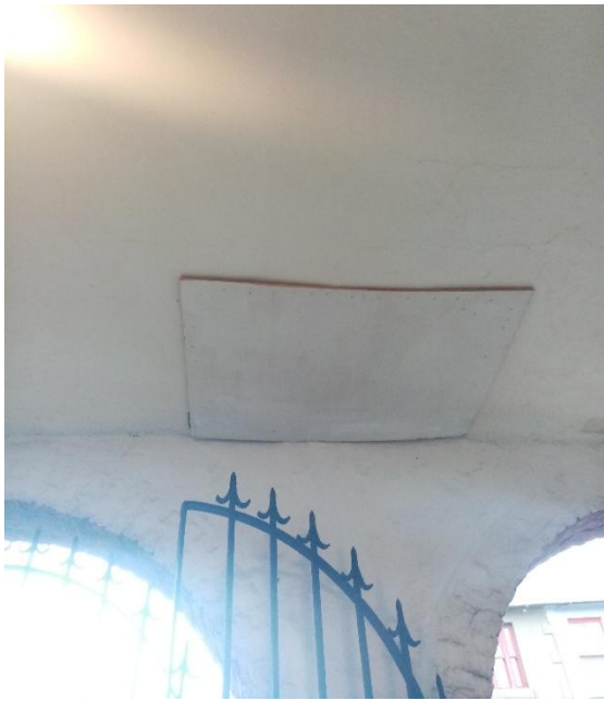
Figure 16: Section of ceiling boarded up which previously collapsed - circled in red in Figure 15
