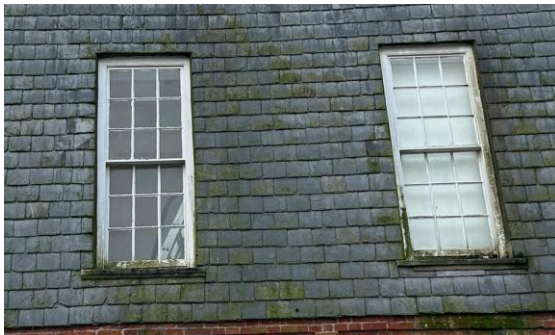
Figure 14: Window on the northeastern elevation with suspected OPC reveals
