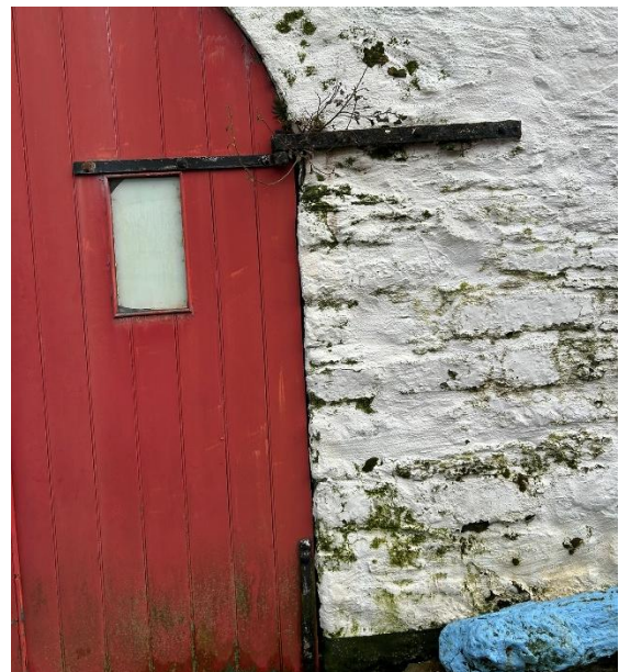
Figure 23: Detail of wrought iron doors hinges
