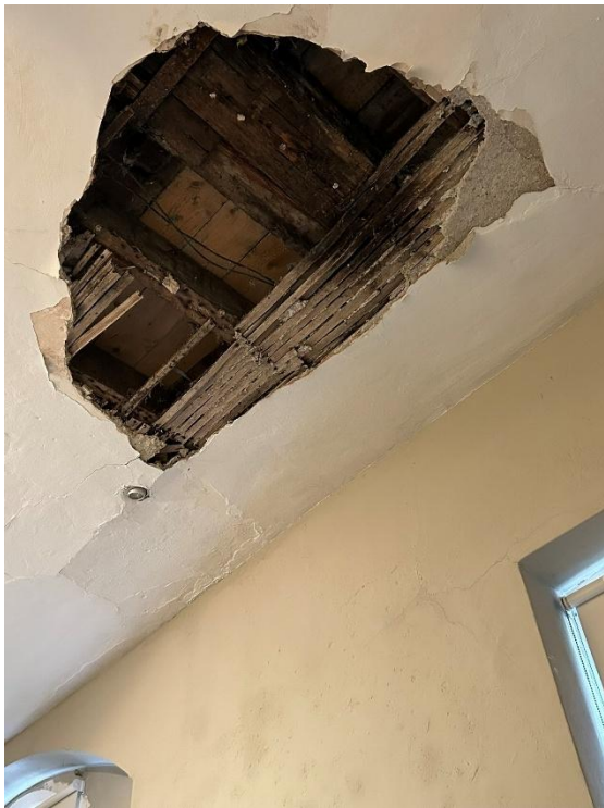
Figure 20: Section of collapsed ceiling in the exhibition space prior to boarding up - circled in red in Figure 9
