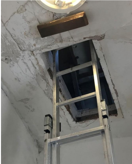
Figure 27: View of attic access hatch
