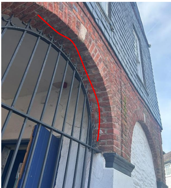
Figure 6: Detail of subject crack highlighted
