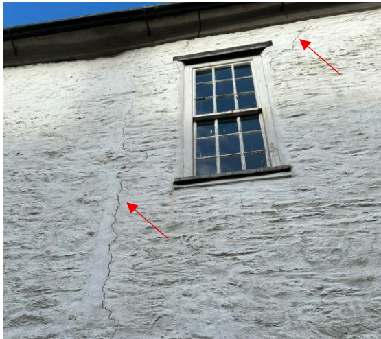
Figure 10: Detail of cracking on southeastern elevation
