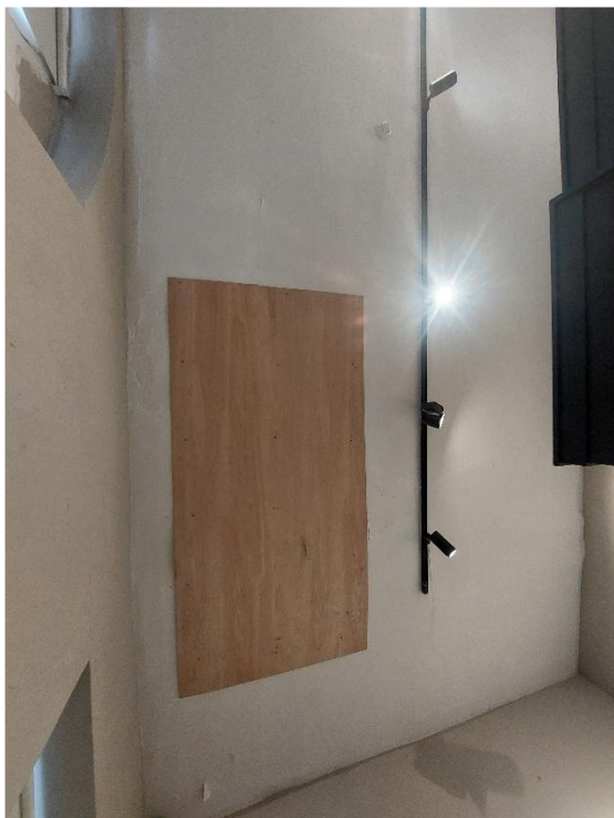
Figure 21: Section of collapsed ceiling in Figure 10 now boarded up
