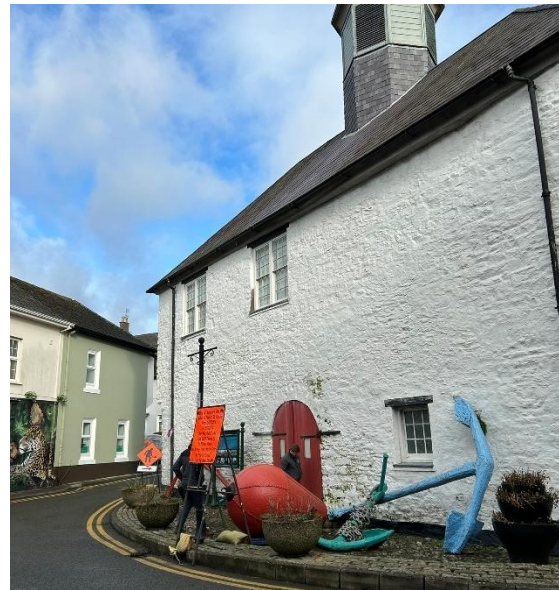
Figure 25: View of southwestern elevation where there is evidence of a broken gutter as observed on a wet day
