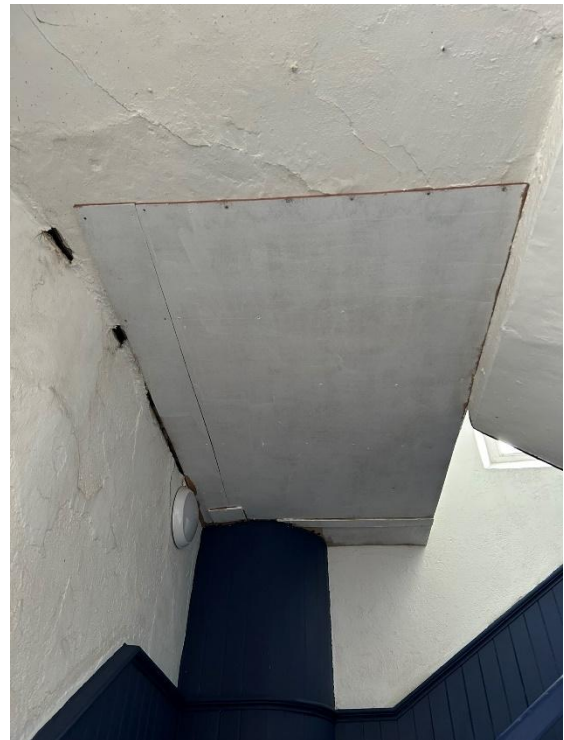
Figure 18: Section of ceiling boarded up which previously collapsed - circled in red in Figure 17
