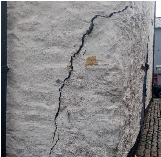
Figure 9: Detail of crack on southern corner
