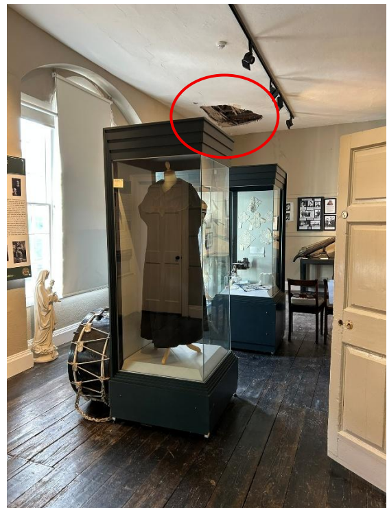
Figure 19: View of First Floor Exhibition space directly above the Arcade looking Southeast
