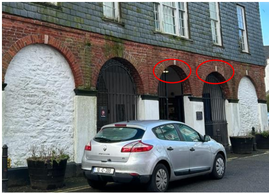
Figure 5: Location of subject cracks highlighted
