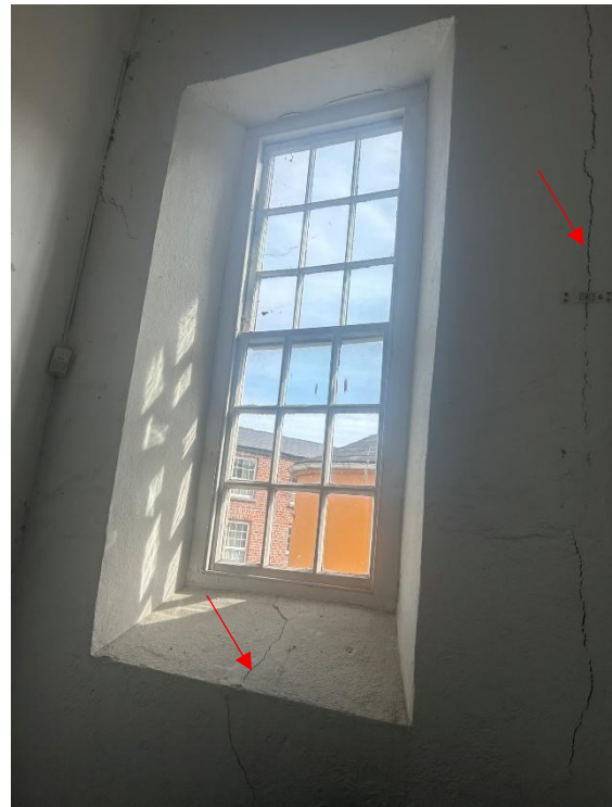
Figure 11: Internal cracks which correspond to the external cracks
