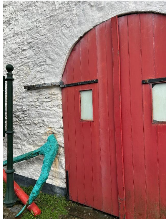
Figure 22: View of Fire Doors and wrought iron hinges
