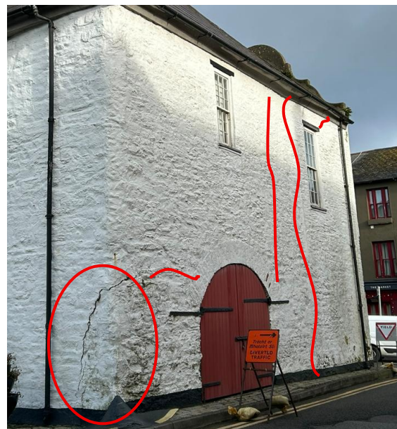
Figure 8: Location of subject cracks highlighted
